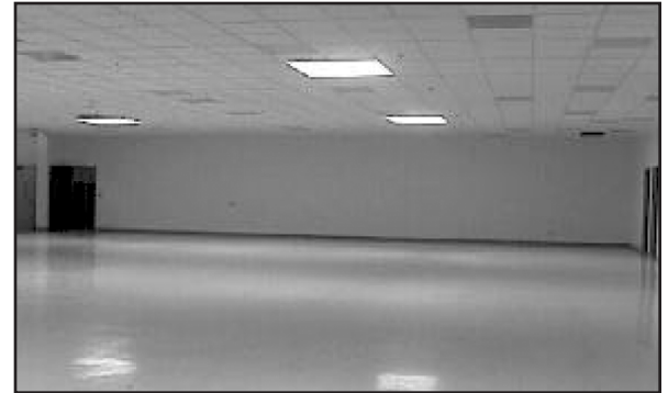
T-BAR CEILING WITH 10' DROPS
